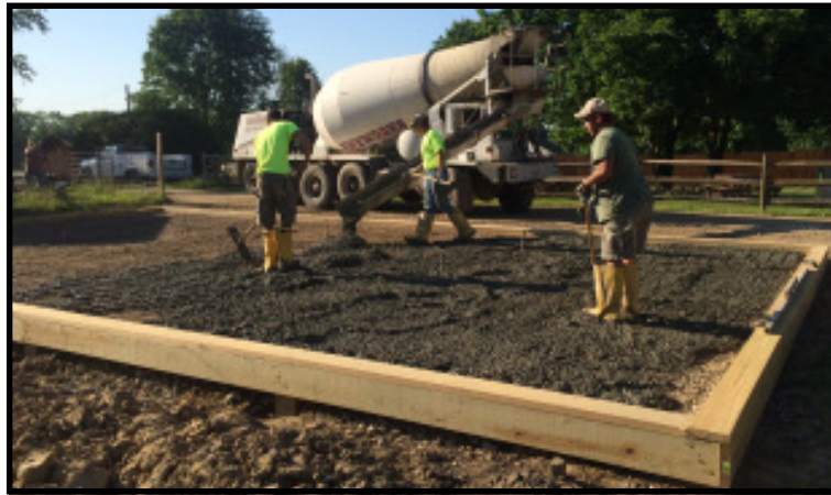
John Rock and his crew filled in the concrete for the floor of the new two-storey multi-purpose building on Saturday, June 7th. On this project, no pigs got loose this time to run through the fresh cement....
