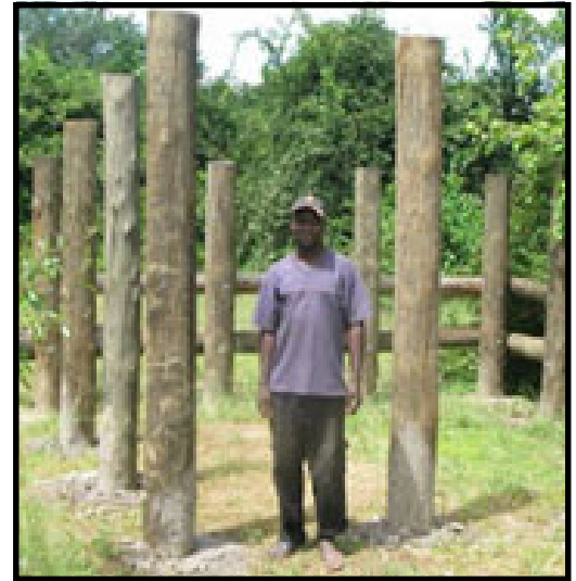
A new shelter in the works.
