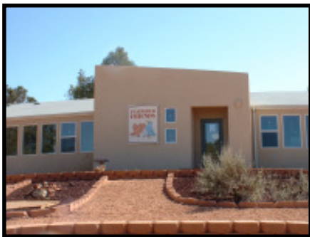
The buildings which housed the dogs, cats and birds were state-of-the-art, and all the grounds were very nicely manicured..
